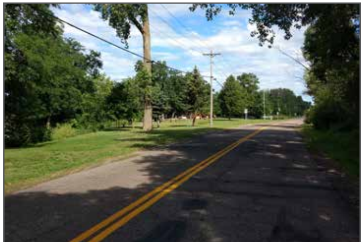
5 Existing conditions of Hugo Road.
