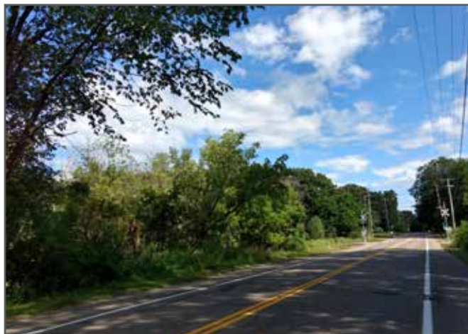
3 The shoulder along Bald Eagle Avenue narrows as the road extends north.
