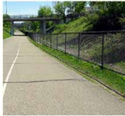
BNSF RR ROW Fencing - 6' Ht. Black vinyl clad chain link
