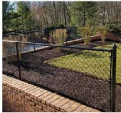
Fall Protection Fencing - 5' Ht. Black vinyl clad chain link on top of retaining walls
