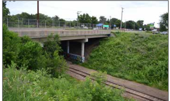
3 Highway 61 bridge crossing over BNSF.
