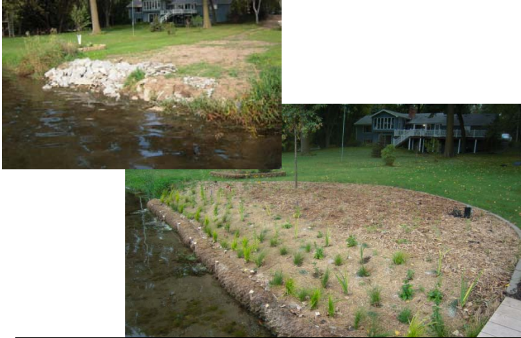
A before and after photo of a shoreline stabilization project completed on Lake McCarron's in Ramsey County, with assistance provided by the RCD.
