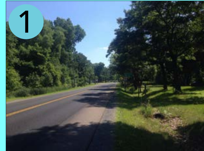
Corridor B has sloping shoulders and drainage swales along Northwest Avenue which would need to be mitigated for trail development.
