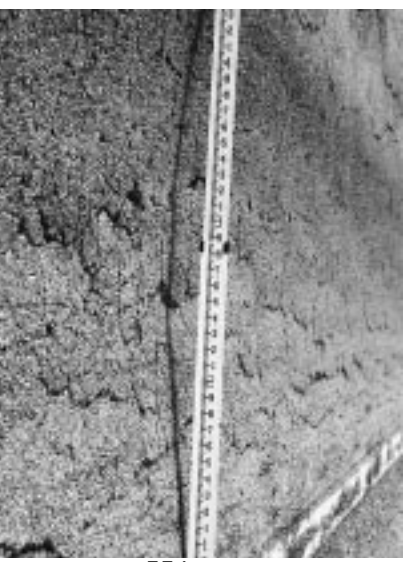
▶ Severe rutting. Strengthen base and reconstruct.
