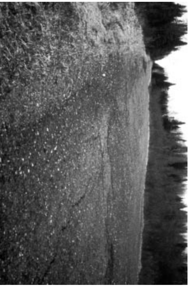
▶ Patches in poor condition, wheelpath rutting. Pulverize, strengthen and reconstruct.
