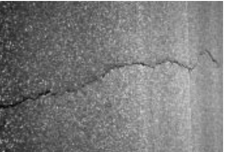
▲ Tight cracks less than \frac{1}{4} " in width.
