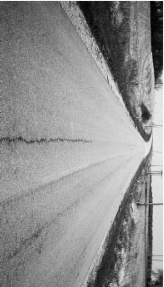
▼ Slight rutting; patch in good condition.
