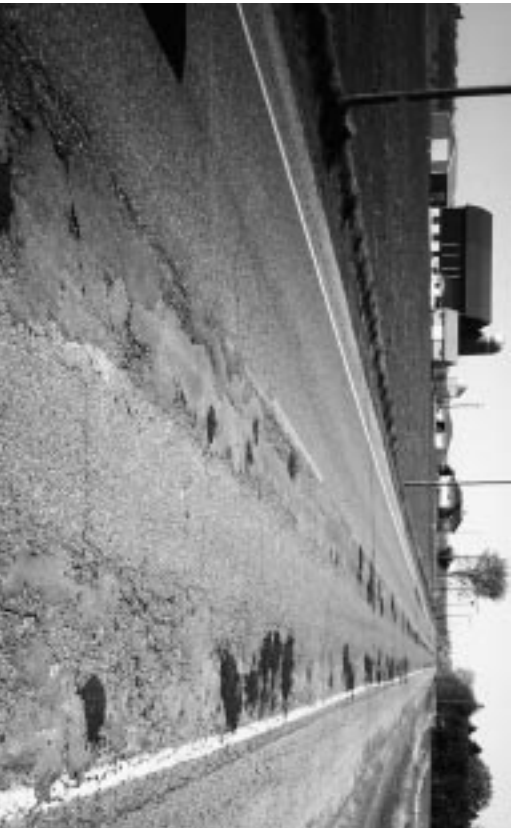
▶ Severe rutting. Strengthen base and reconstruct.
