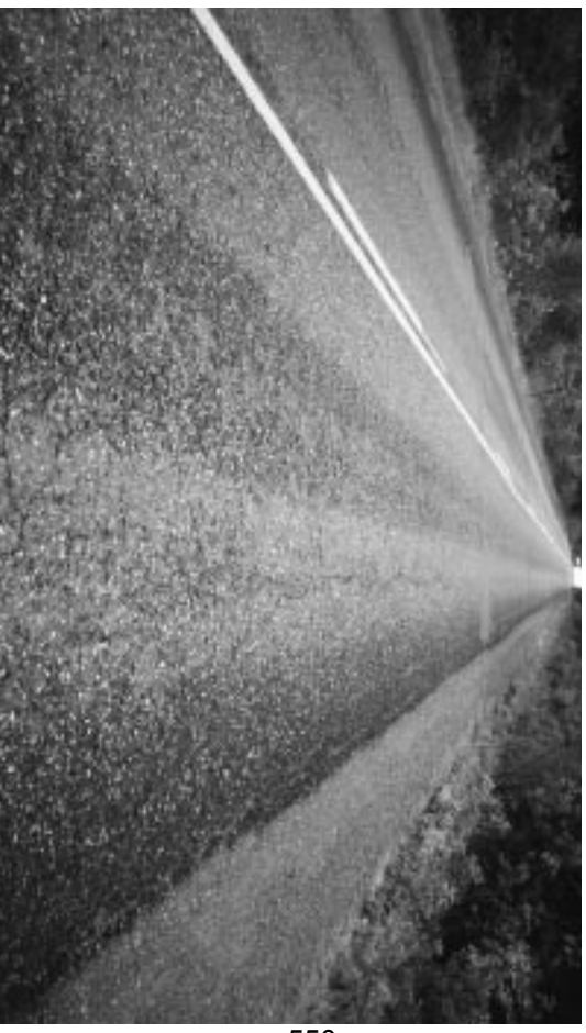
▼ Moderate to severe raveling in wheel paths.
