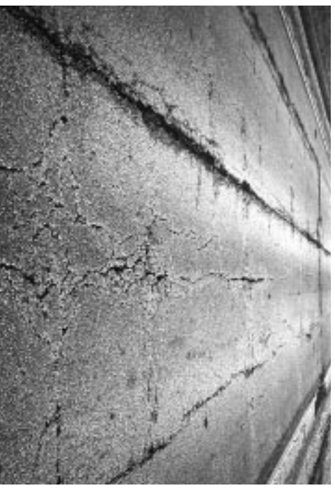
Multiple open cracks at center line, wheelpaths and lane center. ▼
