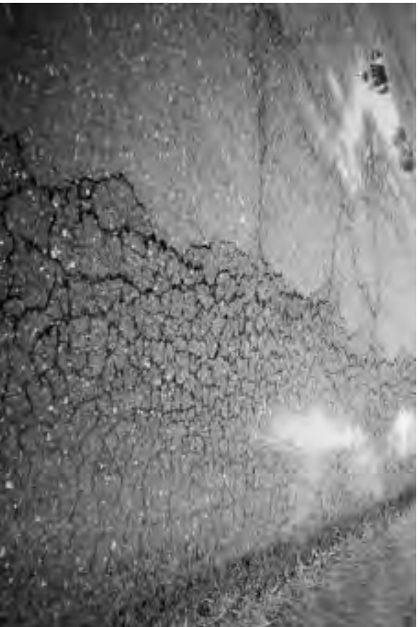
▼ Open raveled alligator cracking with settlement along lane edge most likely due to very soft subgrade.
