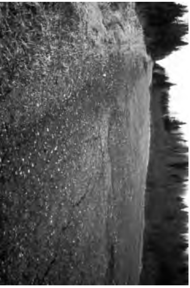
▶ Patches in poor condition, wheelpath rutting. Pulverize, strengthen and reconstruct. ▶ Severe frost damage. Reconstruct.
