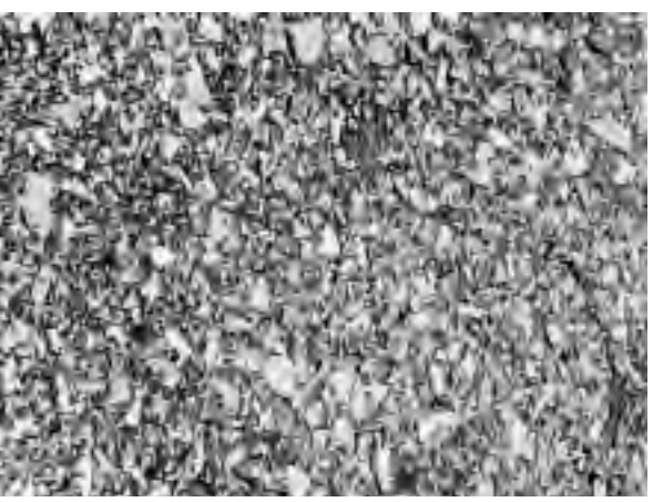
Polished, worn aggregate needs repair. ▶
