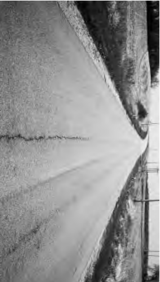
▼ Slight rutting; patch in good condition.
