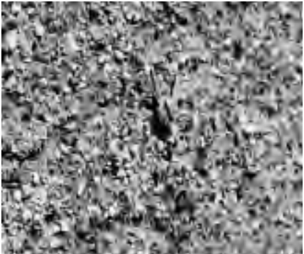
Severe raveling with ▼ extreme loss of aggregate.
