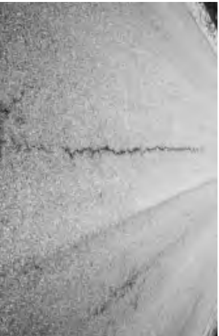
Multiple open cracks at center line, wheelpaths and lane center. ▼
