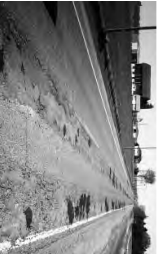
▶ Severe rutting. Strengthen base and reconstruct.
