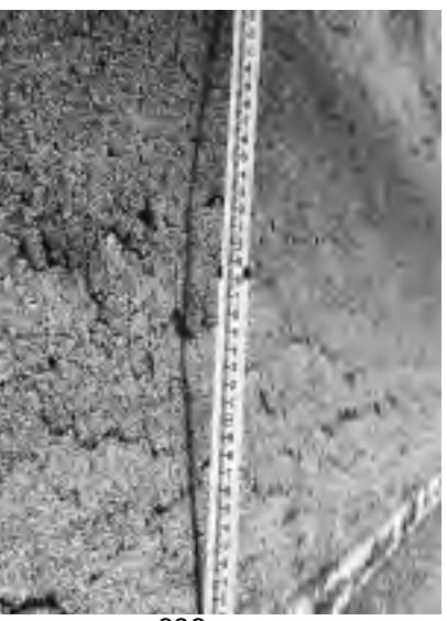
▶ Severe rutting. Strengthen base and reconstruct.
