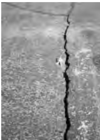
▲ Open crack – 1/2" or more in width.
