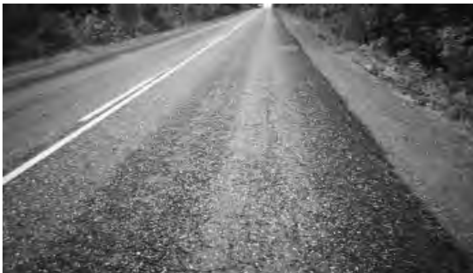
► Moderate to severe raveling in wheel paths.
