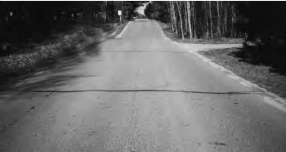
▼ Widely spaced, well-sealed cracks.
