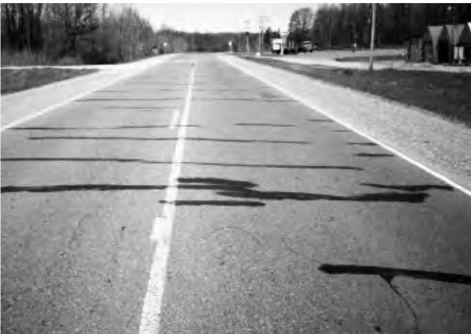
◀ Sealed cracks, a few feet apart.
