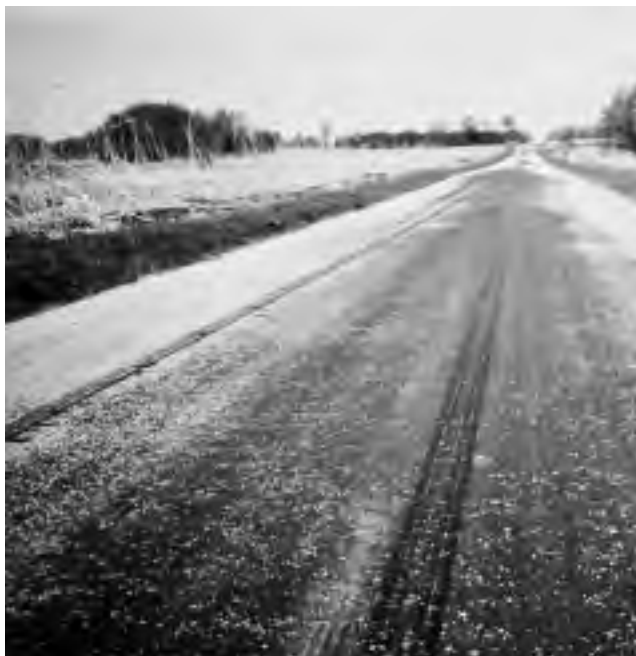
▼ Severe flushing.
