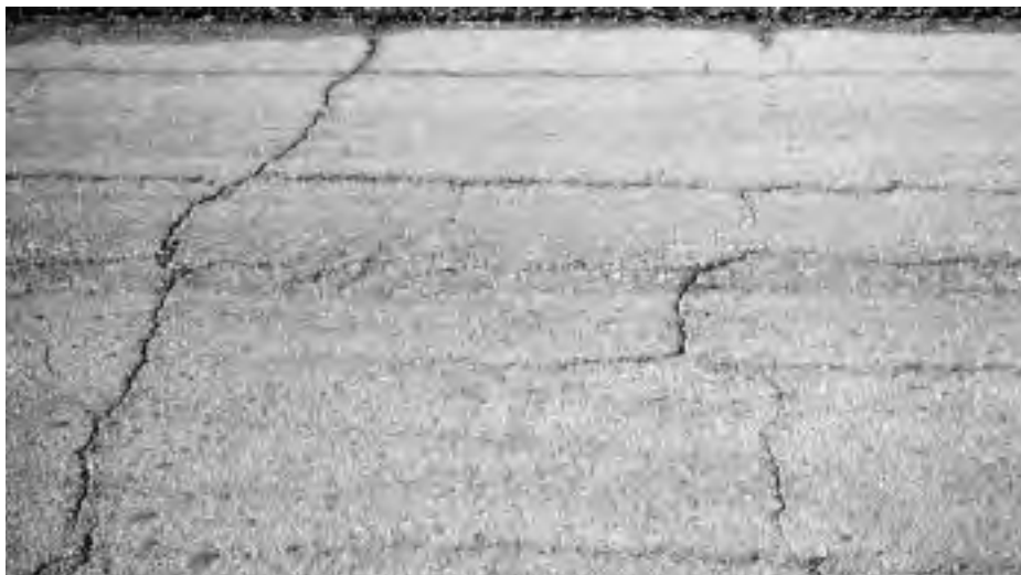
▼ Block cracking with open cracks.
