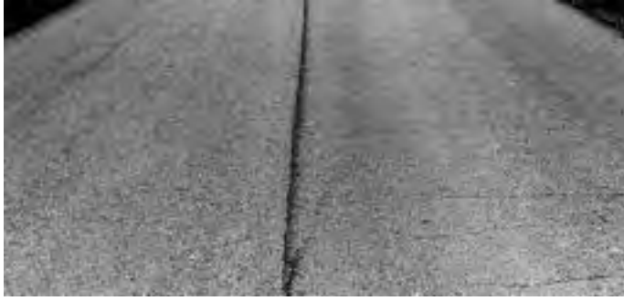
Centerline crack (still tight). ▶
