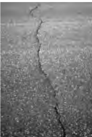
▲ Tight cracks less than 1/4" in width.
