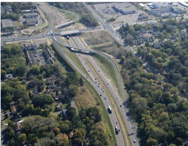
Aerial view of interchange at Hwy 36 and Rice St.
