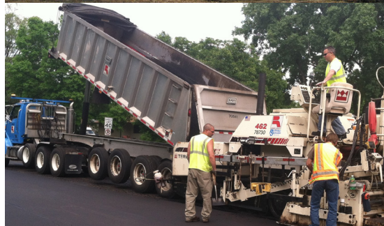
Top Right: Keller Clubhouse construction from 10th fairway. Bottom Right: County maintenance crews improving County roads
