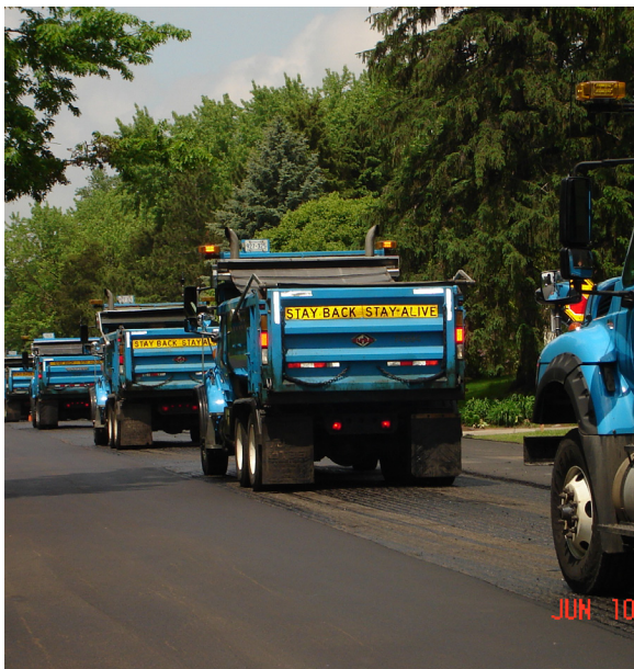
Ramsey County Road Maintenance Crews using County owned equipment to pave Fairview Avenue in Roseville
