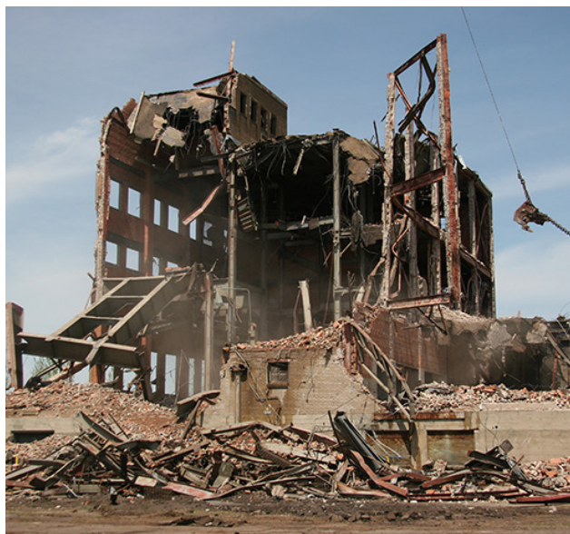
Demolition of the ammunition plant administrative building
