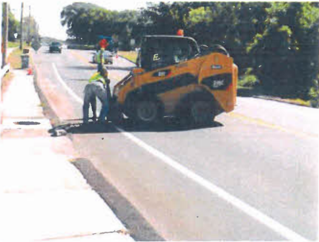
Bobcat operation and direction of crew lead at jobsite.
