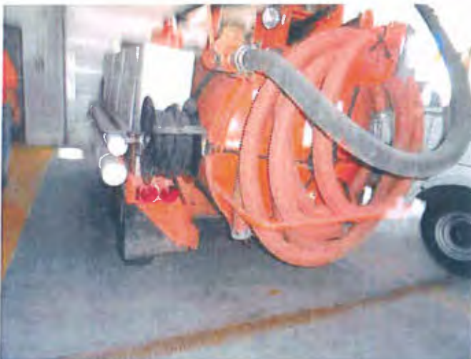
Hoses for vacuum excavator machine (used with gas/utility).
