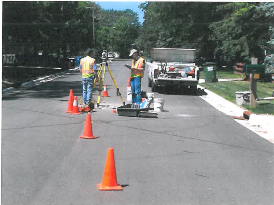
Survey crew setting up at jobsite. Tub of materials can be moved by 2 employees and can weigh between 50-100 lbs.
