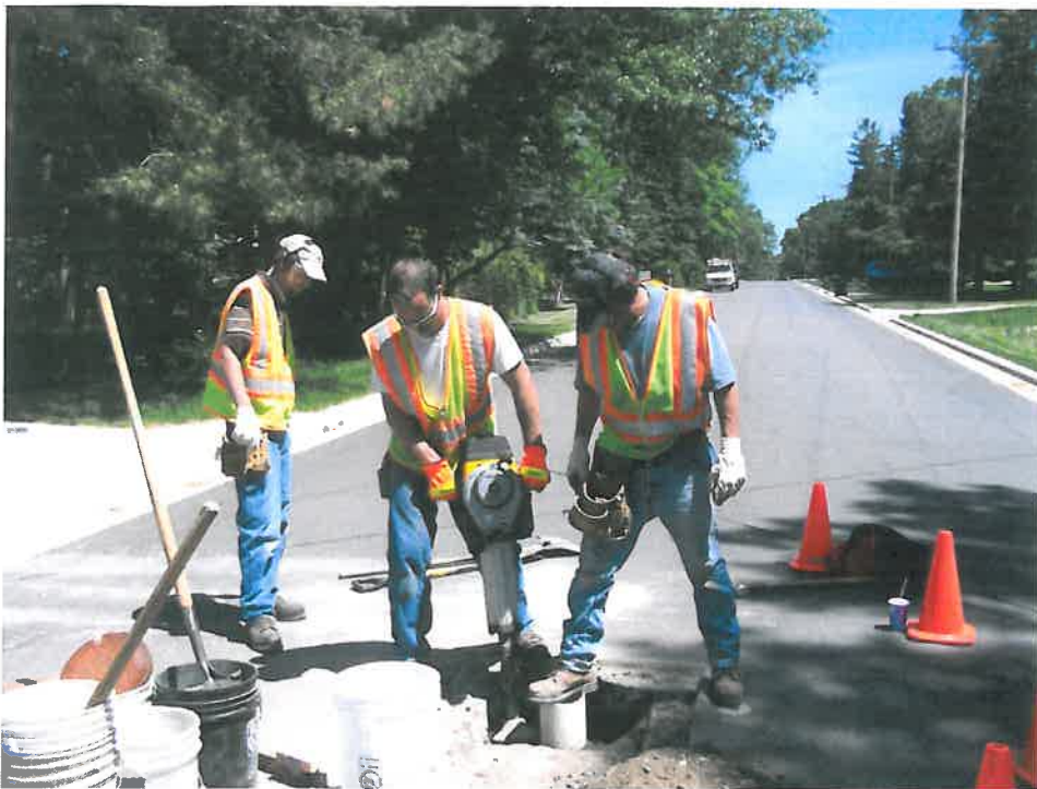
Jack hammer use is rare. Weight is 60 lbs. Firm grip is needed for its operation.
