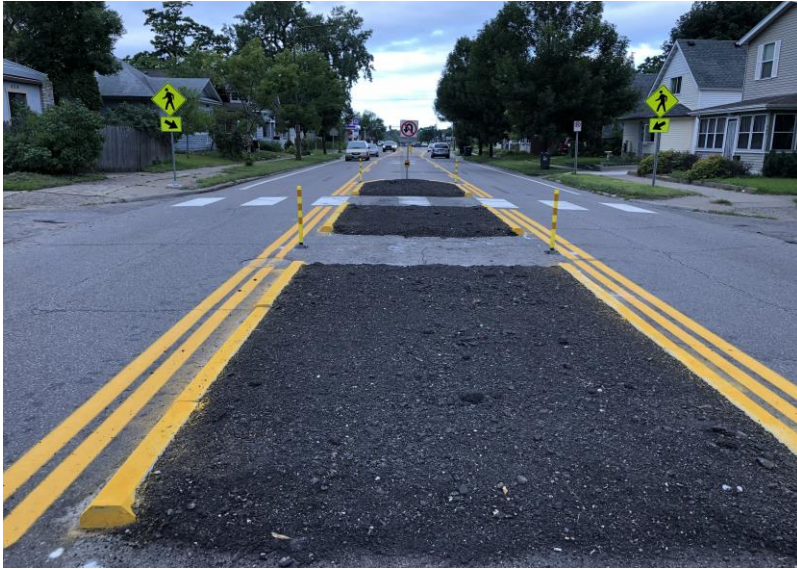
Maryland Ave from Arkwright St to Payne Ave
