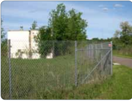
Buildings on the site will be torn down and contamination addressed before the site is available for recreational use.
