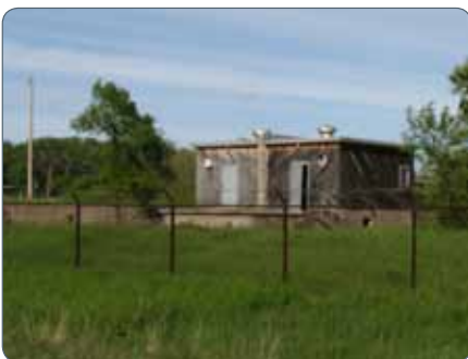
One of the TCAAP structures that will need to be removed from the Rice Creek North Regional Trail Corridor property.
