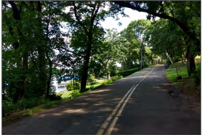
4 No shoulders or separated facilities exist along the narrow stretches of Bald Eagle Boulevard.
