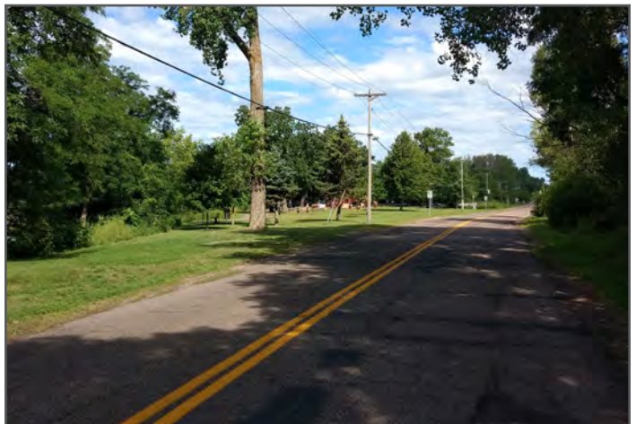
5 Existing conditions of Hugo Road.
