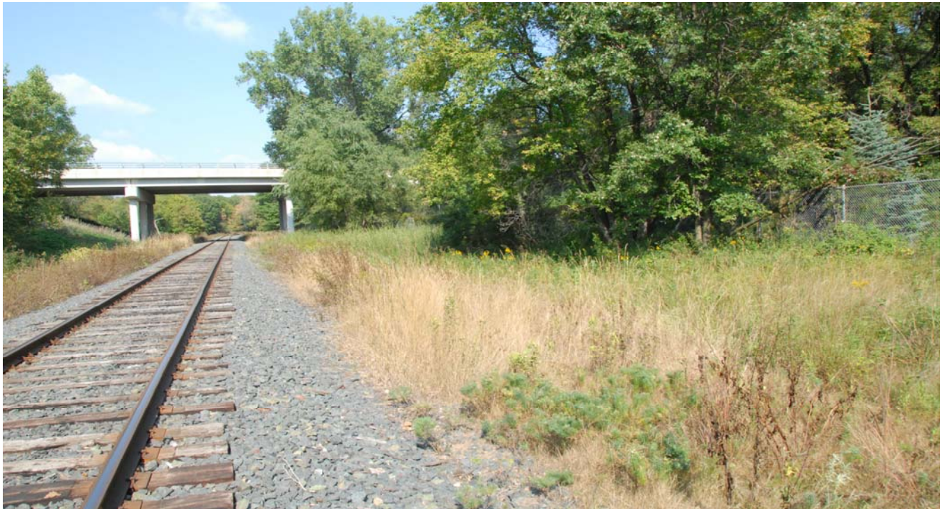
Figure 4 - SPRWS North to Roselawn - Adjacent to Police Canine Training Facility
