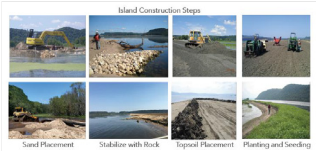
Figure 4: Island Construction Steps (MPA pg. 6)
