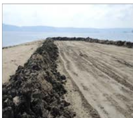
Topsoil Placement
