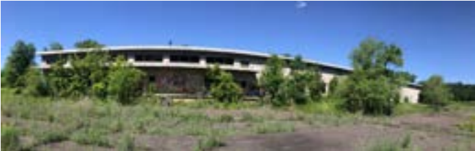
Exterior View of Building 189
