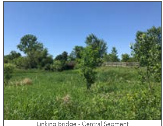
Linking Bridge - Central Segment
