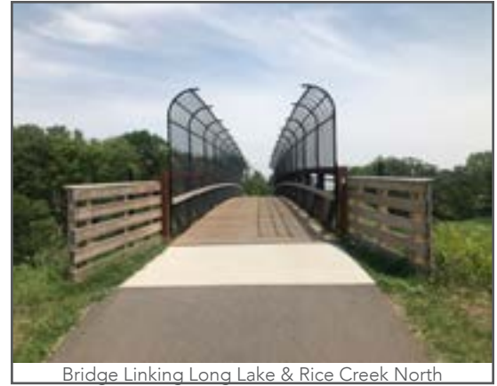
Bridge Linking Long Lake & Rice Creek North
