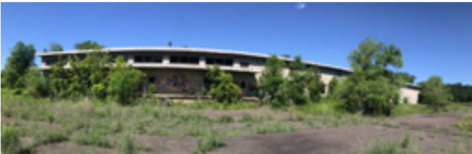
Exterior View of Building 189
