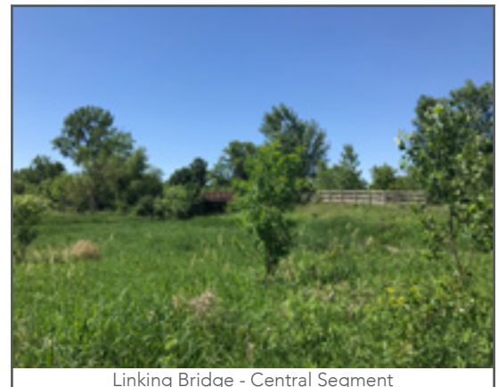
Linking Bridge - Central Segment
