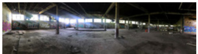
Interior View of Building 189 Point 1, Page 3
