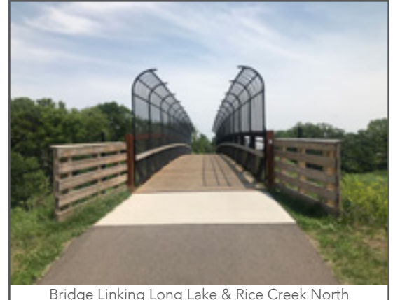
Bridge Linking Long Lake & Rice Creek North
