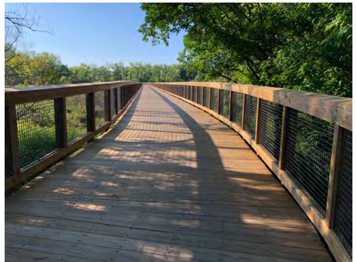
Boardwalk with 42-inch railing.
