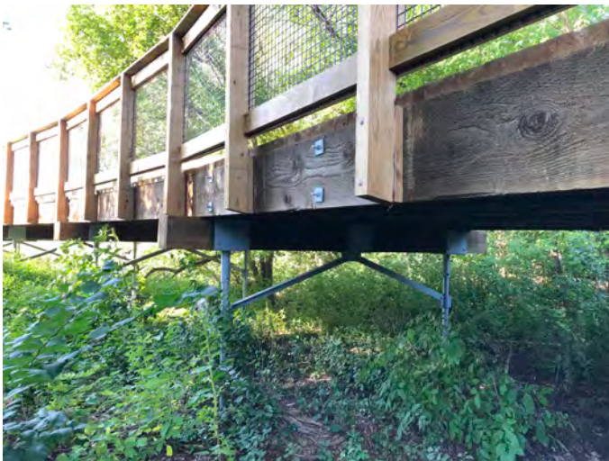
Helical pile foundation.
