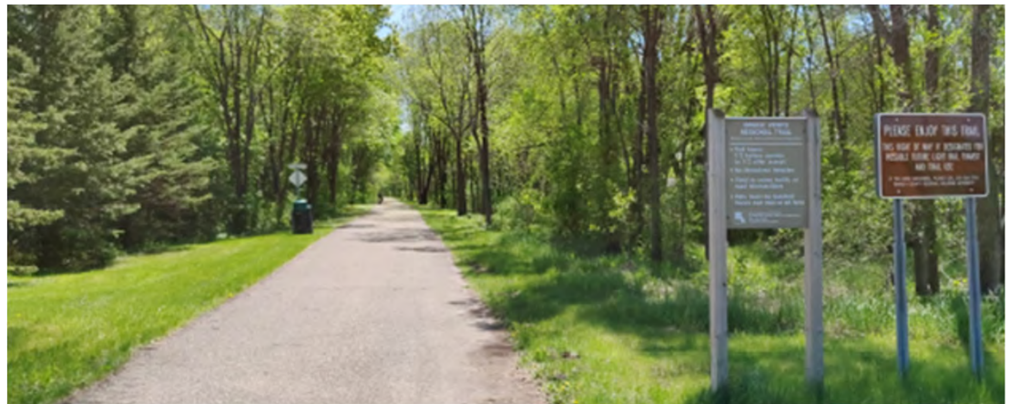
Existing Bruce Vento Trail in Ramsey County rail right-of-way
