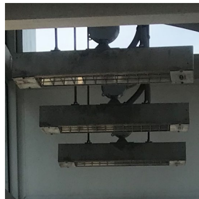
Platform Light & Heaters (A Line Shown)
