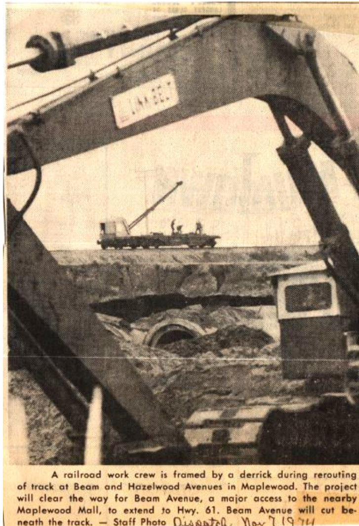
Figure 97. 1974 Saint Paul Dispatch clipping showing construction of the Beam Avenue bridge atop the railroad embankment. The caption notes that “Beam Avenue will cut beneath the track.” 161
