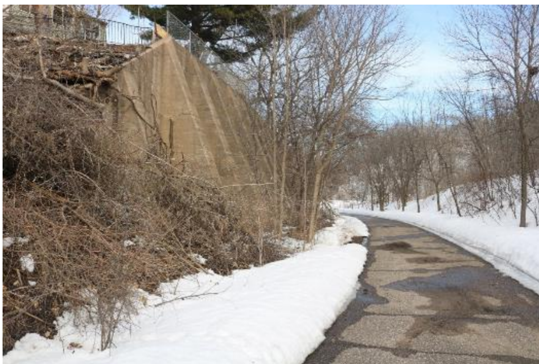
Figure 20. Concrete retaining wall constructed in 1915, located at the rear of 622 Beaumont Street East, view facing north.
