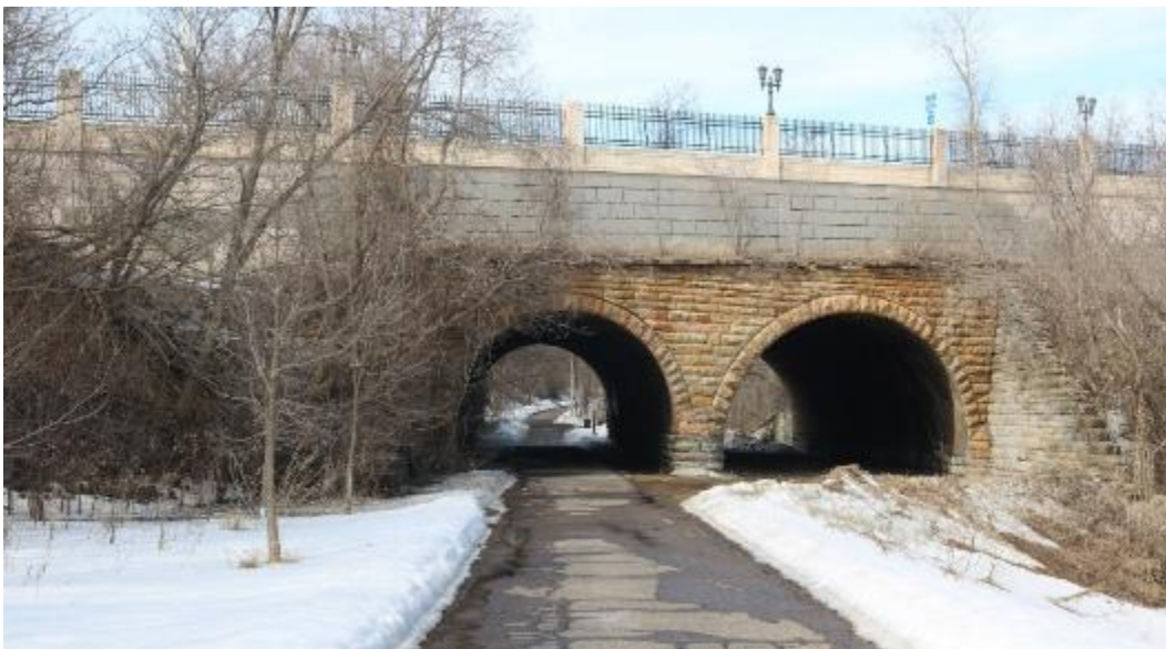
Figure 17. Image of Seventh Street East carried over the LS&M Railroad Corridor Historic District by an 1884 double-arched tunnel (MnDOT Bridge 90386). Note the paved Bruce Vento Trail, which currently utilizes the westernmost tunnel. View facing north.
