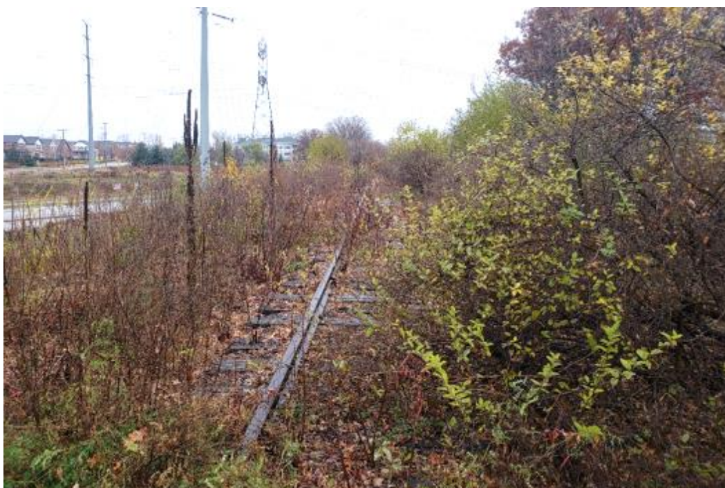
Figure 51. Image of the LS&M railroad roadway north of County Road D, looking south. Note the presence of rails, ties, ballast, and encroaching vegetation. Also note the County Road D vehicular roadway in the background.
