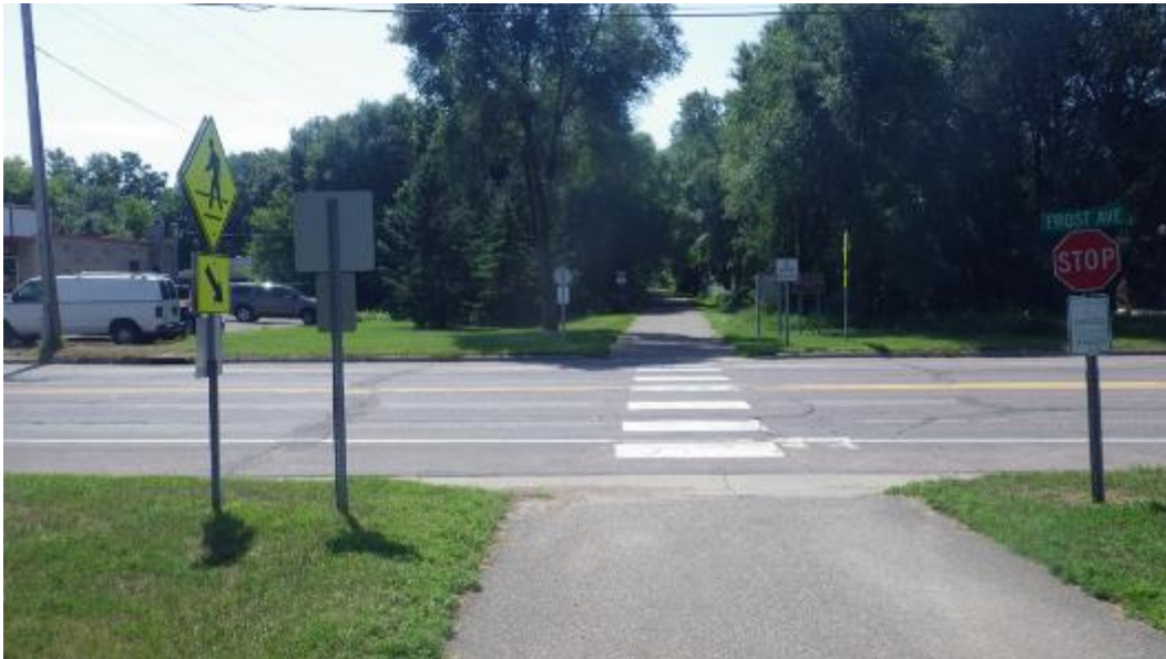
Figure 40. View of modern Bruce Vento Trail facing south at Frost Avenue. Note the minimal embankment and lack of ditched areas.
