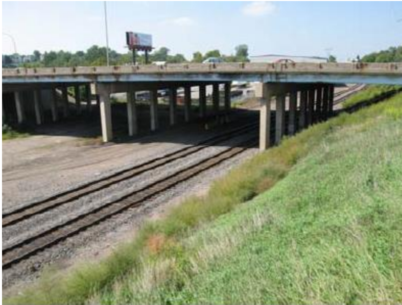
Figure 23. Great Northern Corridor, crossing under I-35E, facing west. 91
