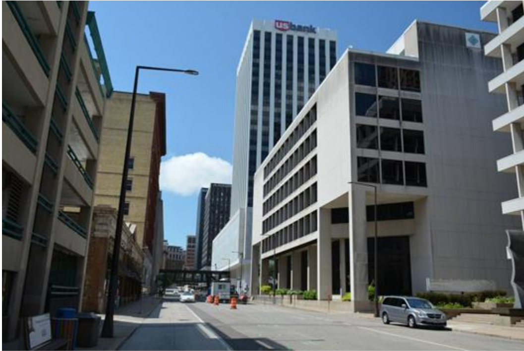
Figure 8. Representative example of the Urban Renewal Historic District’s architecture and streetscape, facing southwest down 5th Street.
