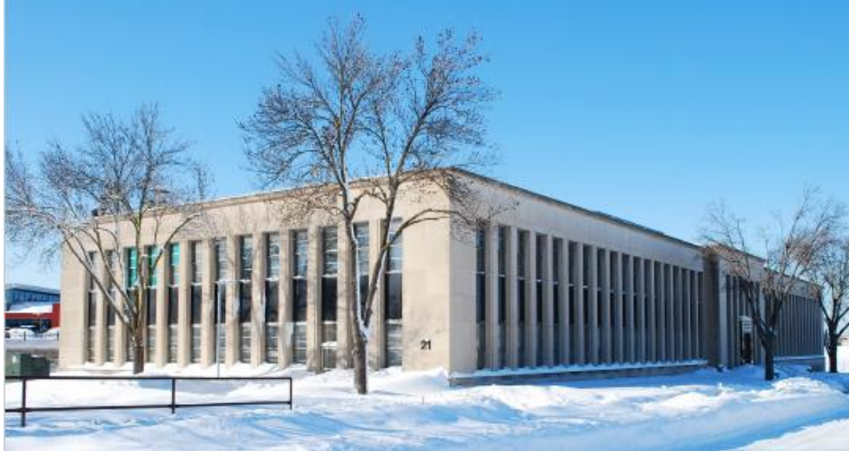
Figure 42. 3M Administration Building, facing southwest. 144
