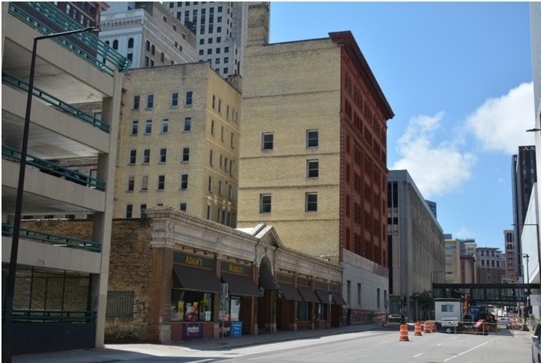
Figure 14. The one-story Endicott Arcade Addition, facing southwest.
