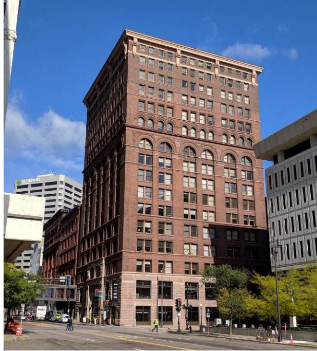
Figure 13. Pioneer and Endicott Buildings, facing north.
