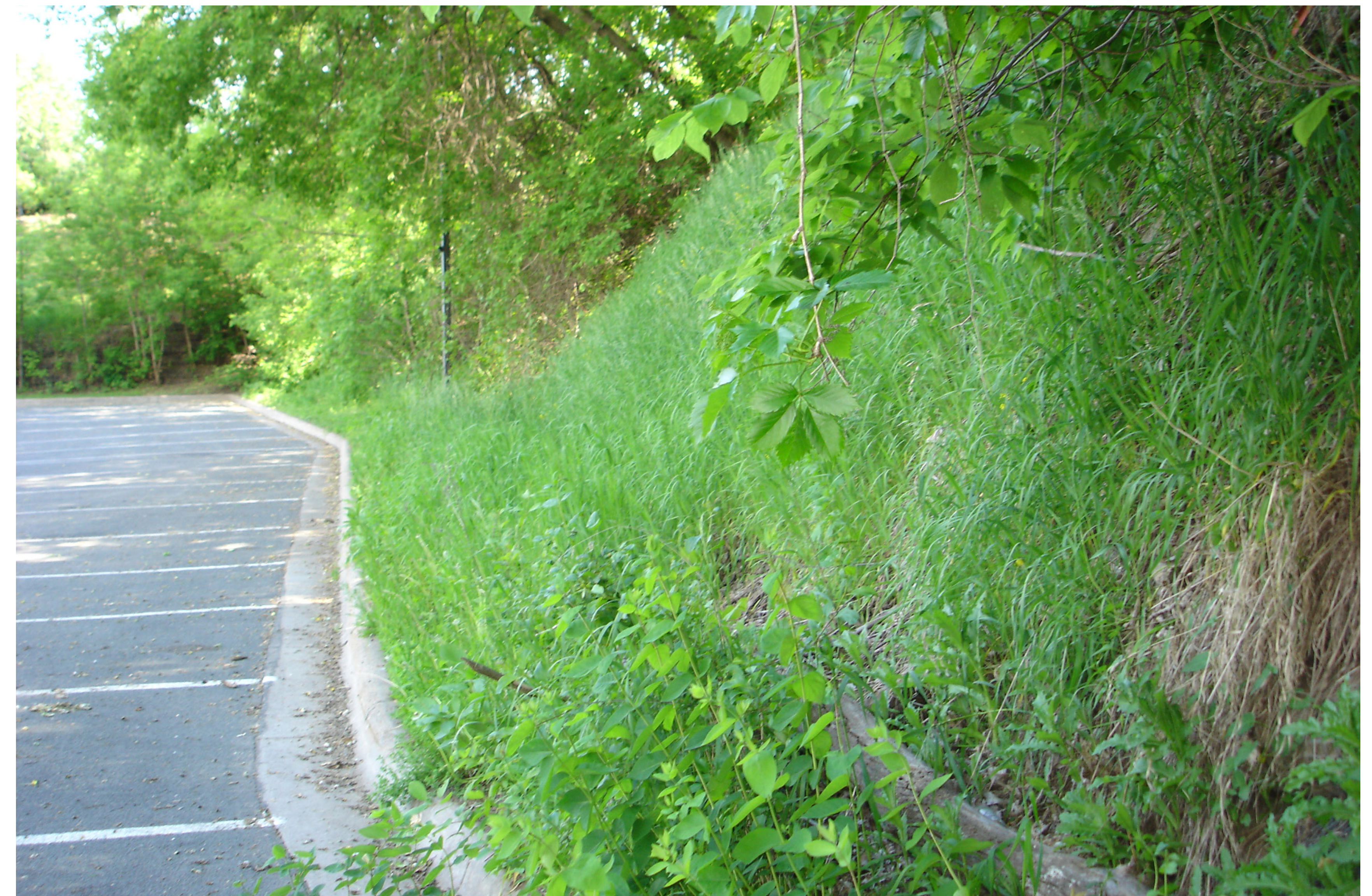
Engineered green slope
