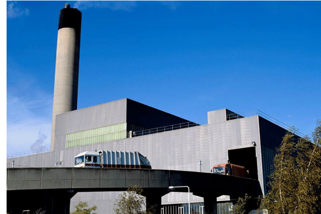
B. Waste-To-Energy Power Plant
