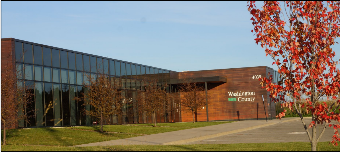
Existing facility, Washington County Environmental Center, MN
