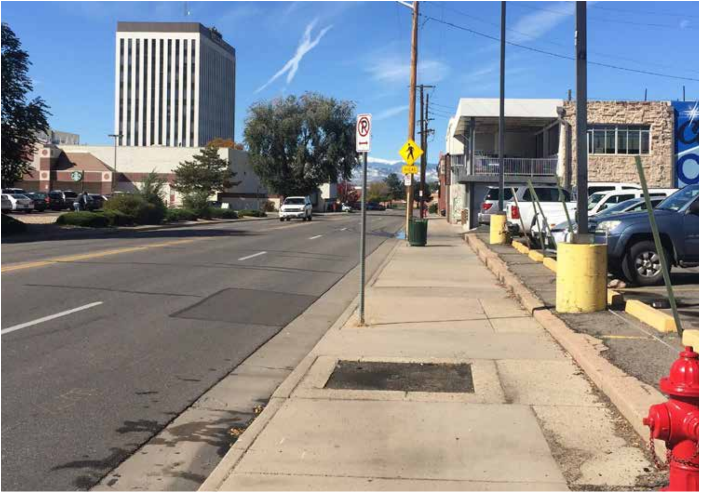
Physical improvements to the corridor should prioritize safety and connectivity for all users, along and across the roadway. (Reema Singh)
