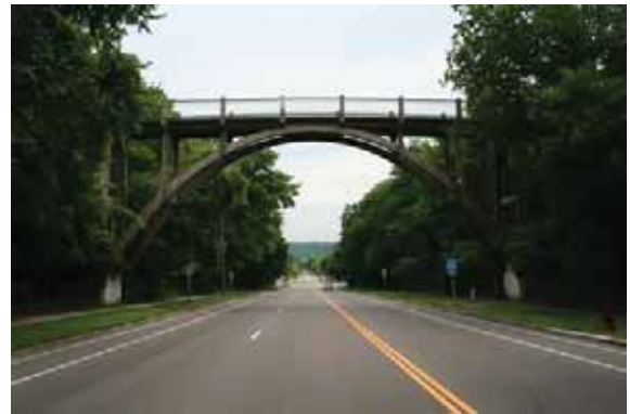
Figure 88: Looking south at the pedestrian bridge over Montreal Avenue, built 1927. Construction of Montreal Avenue required a 40-foot cut through the bluff; the pedestrian bridge connected both sides of the park over the road.
