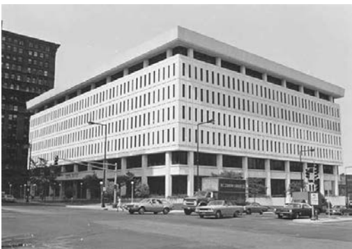
Figure 7: Warren E. Burger Federal Building and U.S Courthouse, 316 North Robert, built 1967. The new federal building was constructed within the Capital Centre redevelopment area, and added another major civic building to Kellogg Boulevard.
