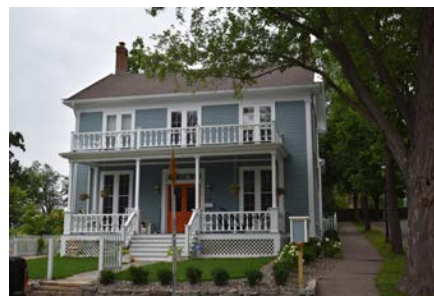
Figure 39: William and Marie Spencer House, 47 Irvine Park, 1860. Renovation of the house began in the 1970s.
