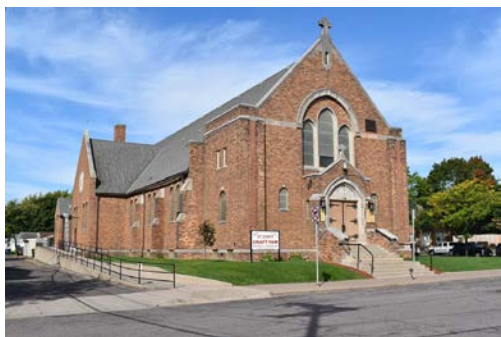
Figure 28: St. Stanislaus Church, 187 Western Avenue.
