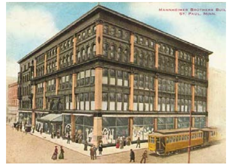
Figure 76: Mannheimer Brothers Building, 115 East 6th Street. (ca. 1910)
