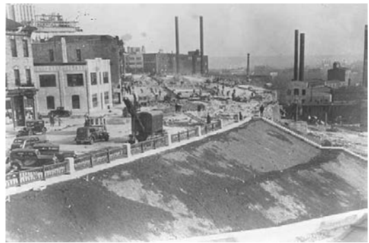
Figure 17: Kellogg Boulevard construction, 1936, looking southeast near Seven Corners. Exchange Street ended at Third Street at left (opposite the stairway) and was not opened due to the steep grade to the Upper Levee. The project created access between Kellogg Boulevard to Exchange by constructing a vehicular ramp in the middle of the boulevard and running down to the lower grade intersection with Eagle Street. (see 1937 aerial, Figure 36, to view the completed construction.) Exchange thus became a vehicular passage to connect Uppertown residents quickly with the improved Kellogg Boulevard.
