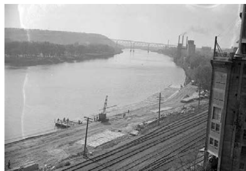
Figure 15: Shepard Road construction west of the Wabasha Bridge, 1949.
