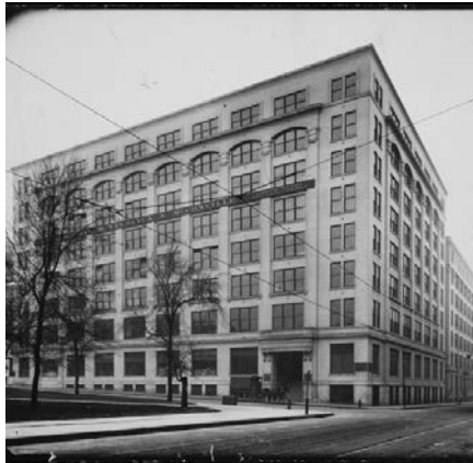
Figure 18: Finch, Van Slyck and McConville Dry Goods Company warehouse at 366 Wacouta, ca. 1911. Facing west toward Smith (Mears) Park, the building was expanded north to Sixth Street in 1923.
