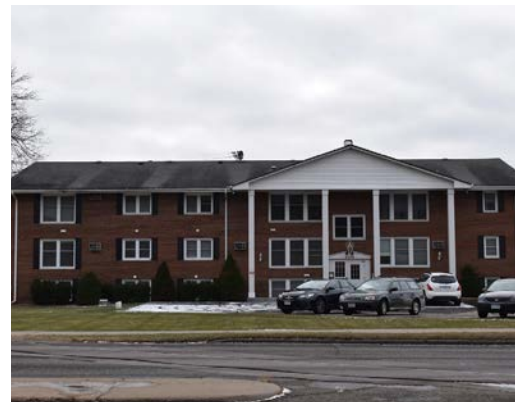
Figure 43: 2390 West Seventh, apartment building constructed 1965 with twelve units. Colonial-style detailing was popular, with the large pedimented portico supported by square columns, an entrance surround with a broken pediment, and shutters accenting all windows.
