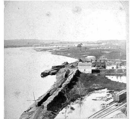
Figure 16: A ca. 1870 view showing the Upper Levee and railroad lines under construction.
