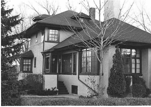
Figure 75: Charles Hausler's Prairie style house, originally along West Seventh but moved to 526 Grace Street in the 1960s.(photo ca. 1974)
