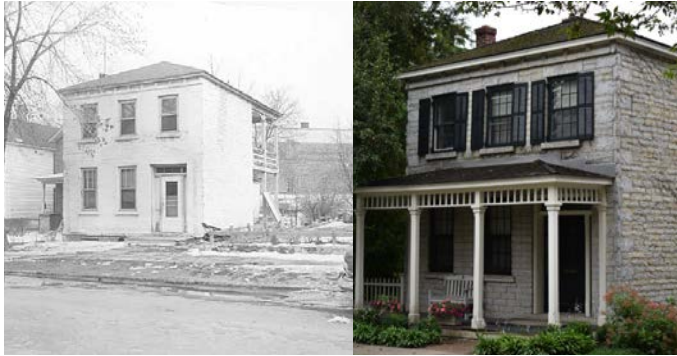
Figures 53-54: Built in 1859 at 314 N. Smith, this limestone dwelling was associated with Joseph and Lucia Brings, who operated a business along West Seventh. The dwelling was moved to a more residential location at 178 Goodrich in 1989 and renovated.
