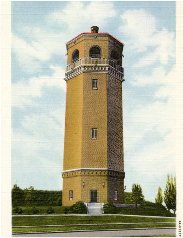
Figure 89: Highland Park water tower, designed by city architect Clarence Wigington, constructed 1929.
