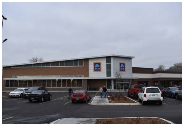
Figure 30: Sibley Plaza, 2401 West Seventh, showing recent renovations and new Aldi store (2019).
