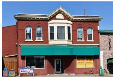
Figure 42: Machovec Building, 997 West Seventh. Machovec's grocery operated at this site for over 100 years and was known for filling grocery orders for Mississippi River barge captains.
