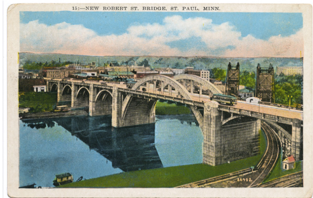
Figure 7: 1927 postcard of the Robert Street Bridge. Built in 1926, the new bridge replaced the 1884-85 structure with a Moderne design of reinforced-concrete arches, and the rainbow arch ribs that created a distinctive profile and gateway into downtown St. Paul.
