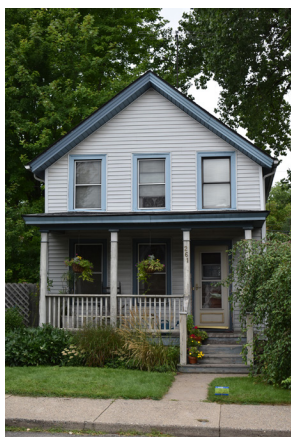
Figure 33: John O'Donnell House, 261 Banfil Street, built 1857.
