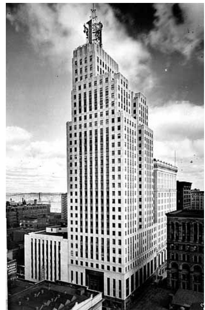
Figure 37: First National Bank, 332 Minnesota Street, 1931 was the City’s tallest building for several decades, crowned by a red neon “1 st ” dominating the skyline.
