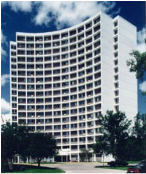
Figure 44: Montreal Hi-Rise, 1085 Montreal Avenue, senior housing completed in 1970.
