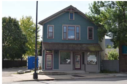
Figure 39: Wasika Building, 974 West Seventh, former location of the Fort Road/West Seventh Federation offices.
