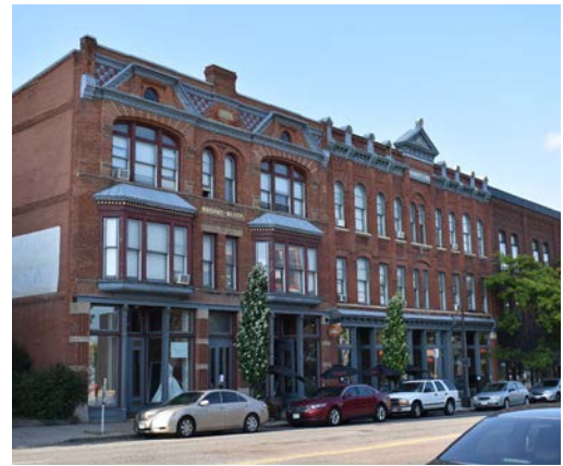
Figure 31: The Rochat-Louise-Sauerwein Block, 261-277 West Seventh, constructed between 1884 and 1895, represented some of the early commercial blocks that began to replace the large older dwellings that previously lined West Seventh. The blocks contained first floor, cast-iron storefronts, with elaborate Queen Anne-style detailing on the upper levels that housed flats and meeting rooms.
