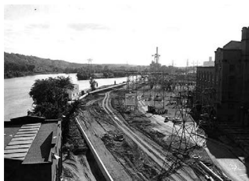
Figure 16: Shepard Road construction near the Northern States Power plant, 1959.
