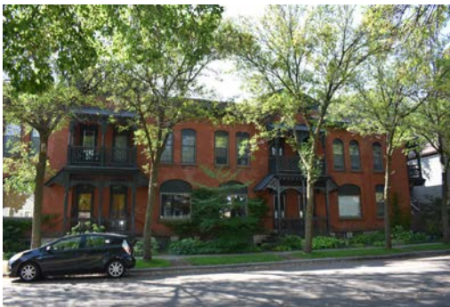
Figure 52: The brick Gardner Rowhouse, 89-97 Leech Street, built 1891, displayed the Queen Anne style with its decorative entry porches and second level balconies.
