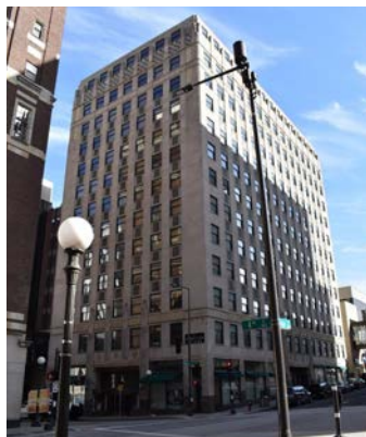
Figure 36: Minnesota Building, 46 Fourth Street East built 1929
