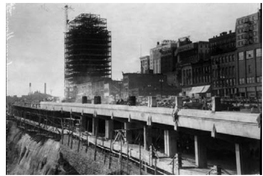
Figure 15: Construction of Third Street improvements, 1931. Second Street ran under the upper level where the Third Street Esplanade would be constructed. The Ramsey County Courthouse and St. Paul City Hall is under construction at the intersection with Wabasha Street.
