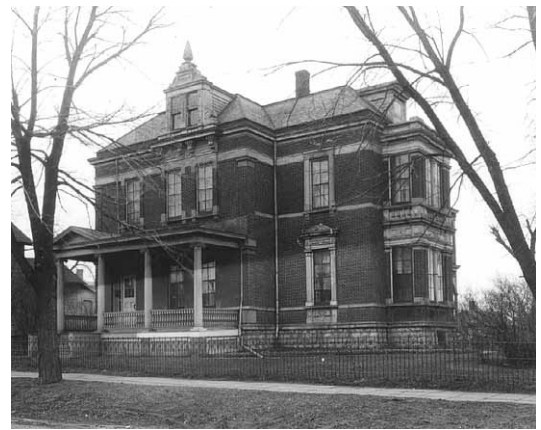
Figure 26: Funk Residence, 398 Duke Street, built 1887. Melchoir Funk operated Funk Brewery, which continued until 1901, at Duke and Palace streets. (1937)
