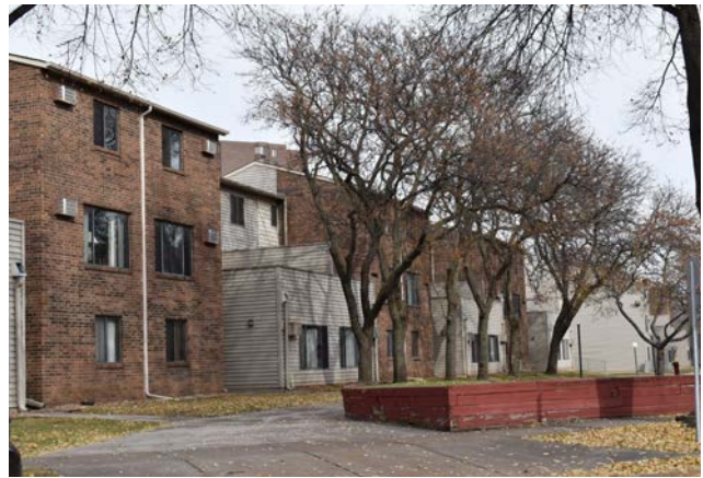
Figure 36: The St. Paul Housing and Redevelopment Authority cleared the trapezoid-shaped block along West Seventh from Sherman to Forbes for a new housing project in the 1970s. Some houses on the block were saved and moved to other nearby locations, while other buildings were razed. The Sherman-Forbes project, designed by Stanley Fishman Architects, Inc. included units that faced inward around a central courtyard with parking lots on the outer edge next to streets.
