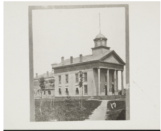
Figure 5: Ramsey County Courthouse, built 1851 between 4th and 5th, Cedar to Wabasha.
