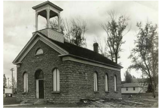
Figure 58: The 1887 limestone Mattocks School at Randolph and Snelling, which served students in Reserve Township. The building was moved to Montreal and Snelling, near Highland Junior/Senior High School in 1964.
