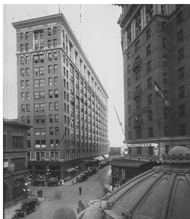
Figure 27: The Lowry Medical Arts Building, 358 St. Peter Street, built 1911-12, was constructed about the same time as the new St. Paul Hotel across the street.
