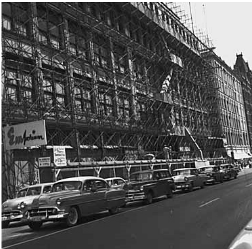
Figure 2: Emporium undergoing renovation, ca. 1958.
