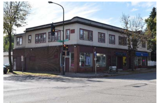
Figure 83: 866 Randolph is a typical commercial and flats building from ca. 1920 on a streetcar intersection corner.
