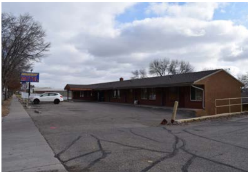
Figure 32: Highway Motel at 2152 West Seventh, 2019. The motel was constructed in 1958 as six units.
