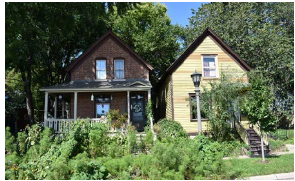
Figure 61: Housing for worker's families tended to be one- and two-story dwellings, with both wood frame and brick exterior finishes. These front-facing gable dwellings were constructed along Butternut Avenue, a neighborhood that grew up near the Banholzer Brewery by the 1880s.
