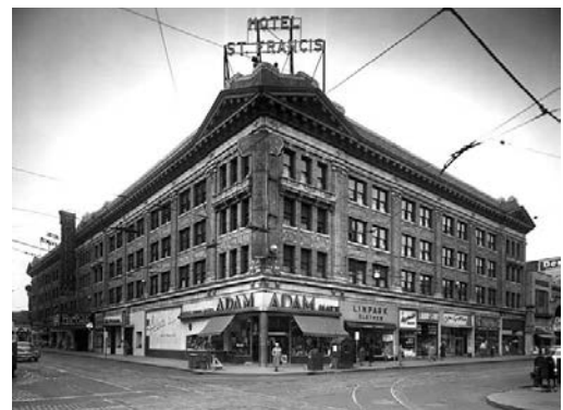
Figure 25: Hotel St. Francis, 9 West Seventh, built 1916. The hotel contained the New Palace Theatre along Seventh (now Seventh Place), which was renamed the Orpheum by the time of this 1953 photo. The cross street on this photo is Wabasha.
