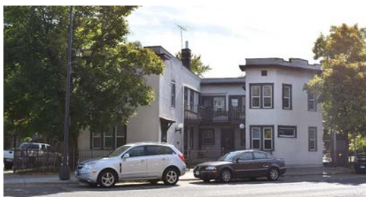
Figure 81: 462 West Seventh is a courtyard-style, stucco apartment building from 1922.
