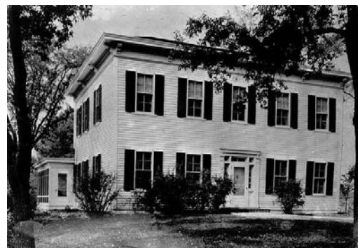
Figures 56-57: One of the earliest houses built in Reserve Township, the 1860s William Davern house showed the Italianate style as applied to a rural dwelling (top photo). In an early example of respecting the historic style, the 1929 addition was so skillful that it appears the entire house was original to the 1860s.
