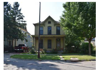
Figure 50: George Krech House, 55 Wilkin Street, constructed 1880.
