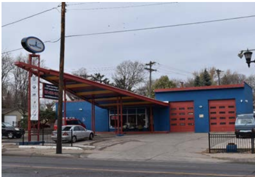
Figure 31: Now Van-Go Auto, this ca. 1959 gas station retains its projecting “space age” canopy.
