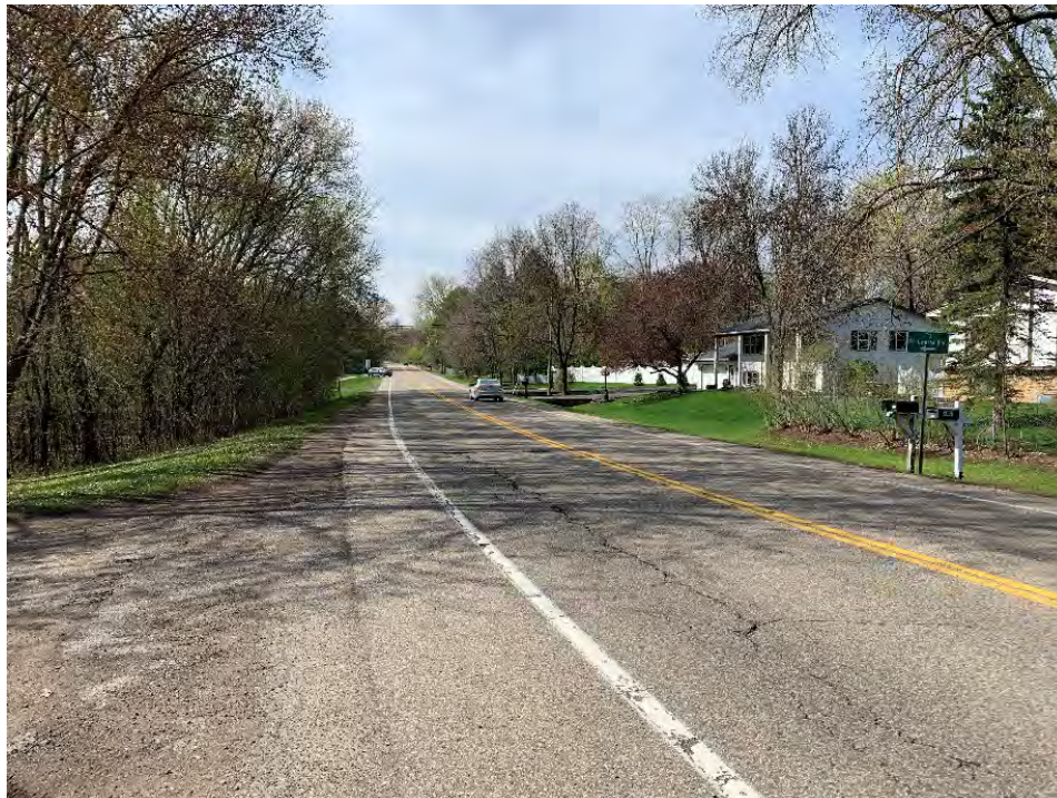
Existing roadway configuration along the northern part of the Victoria Street corridor.
