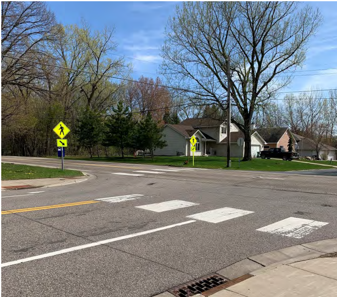
An uncontrolled pedestrian crossing over Victoria Street at W County Rd D.
