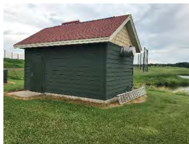
Pump house and station controls
