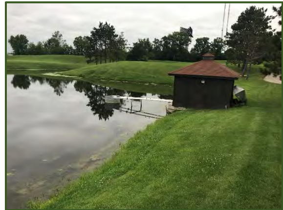
Older pump house and controls – could use an upgrade of more reliable pump equipment rated for golf applications
