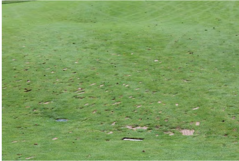
Above -The unintended fairway collection area on the 14th hole. The catch basin is undersized for the drainage area, and typical of the drainage system
