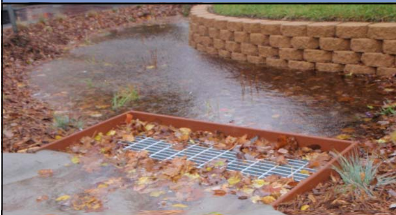
One of 3 Crooked Lake Curb Cut Rain Gardens 3 Months After Installation in 2010
